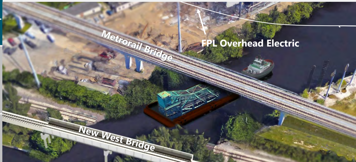
Float Out Bascule Demolition
