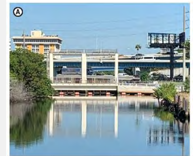
SFWMD S-26 Control Structure
