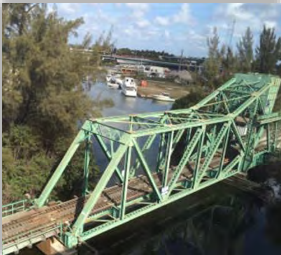
Existing Single Track Bascule Bridge
