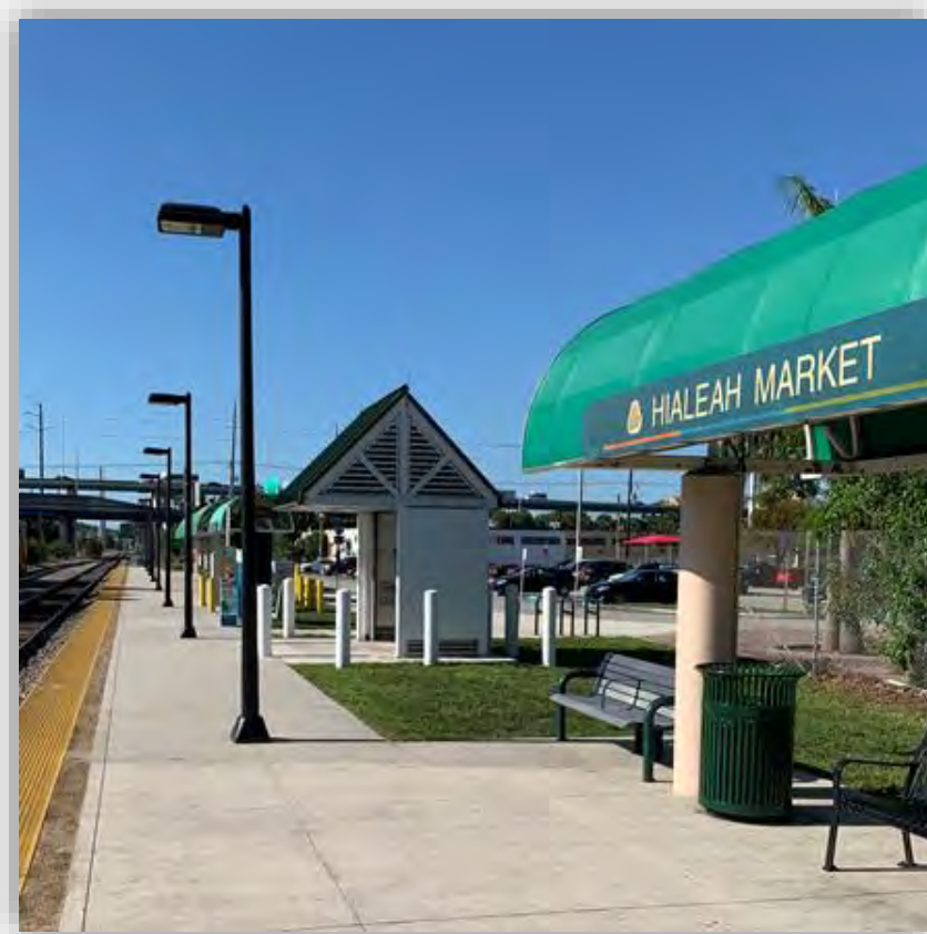
Existing Station – West Side Platform
